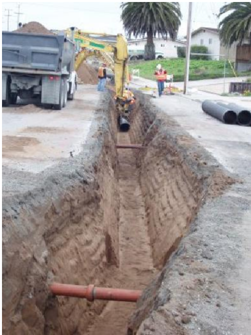
CRESCENT AVENUE CONSTRUCTION #3
