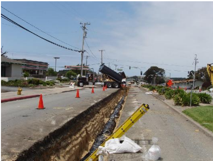
RESERVATION ROAD CONSTRUCTION #1
