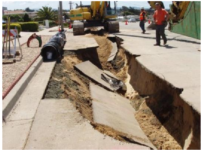
CRESCENT AVENUE CONSTRUCTION #2
