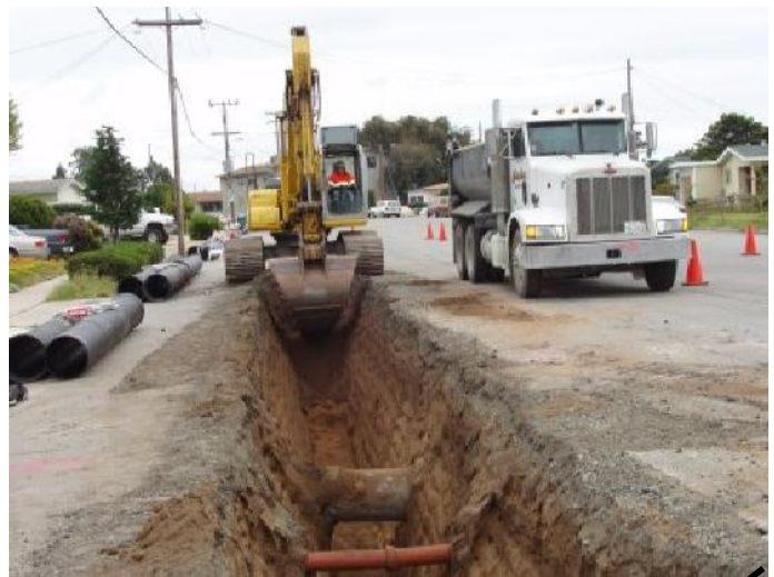
CRESCENT AVENUE CONSTRUCTION #4
