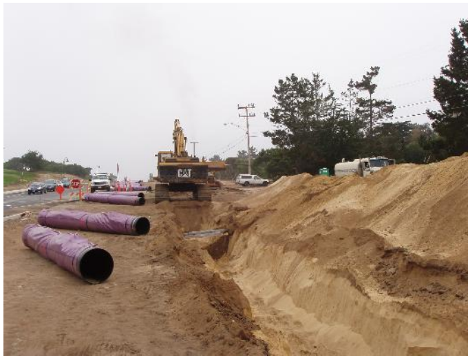
GENERAL JIM MOORE BOULEVARD CONSTRUCTION #1
