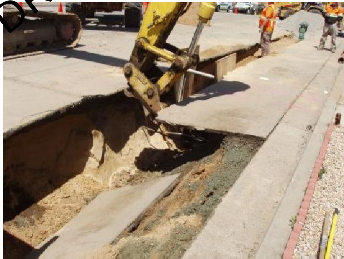
CRESCENT AVENUE CONSTRUCTION #1
